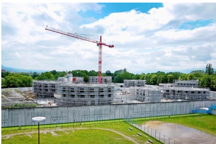
Construction de CURABILIS, TdG 03.04 2014, Image : Pascal Frautschi
